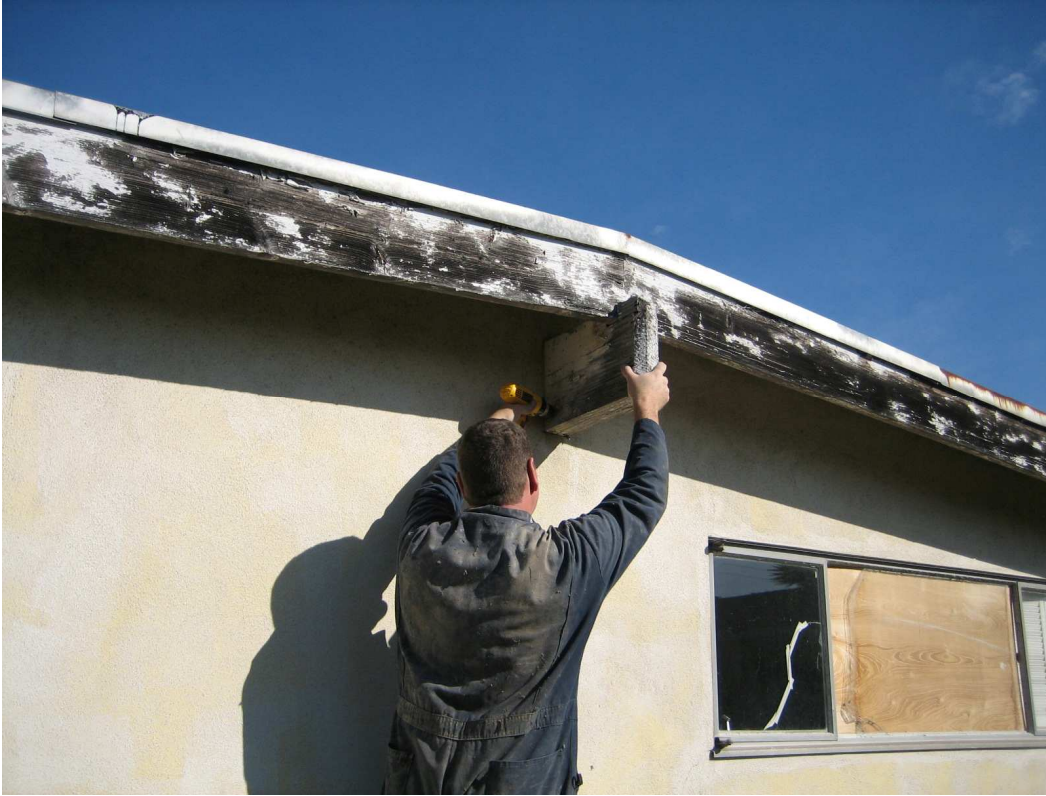
Figure 3. Example of drilling a board infested with drywood termites before Treatment; location Torrance, CA. Included in image is M. Red, Clark Pest Control.
